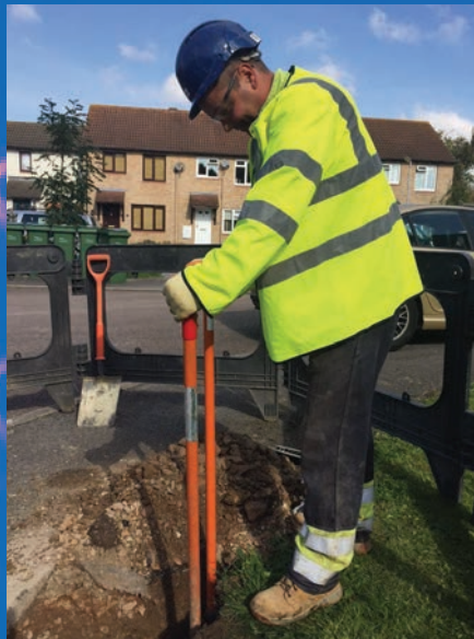
Picture 1; the excavation team digs the footpath
