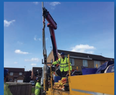
Picture 3; the Hiab removes the redundant lamp column
