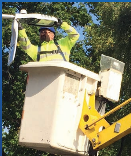
Picture 5; the power is connected. The lighting column is fully functional.
