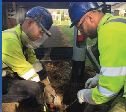
Picture 2; the connection team makes sure the live cable is safely capped
