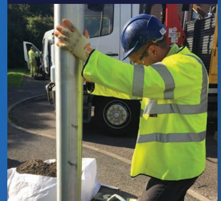
Picture 4; a new replacement steel lamp column is erected
